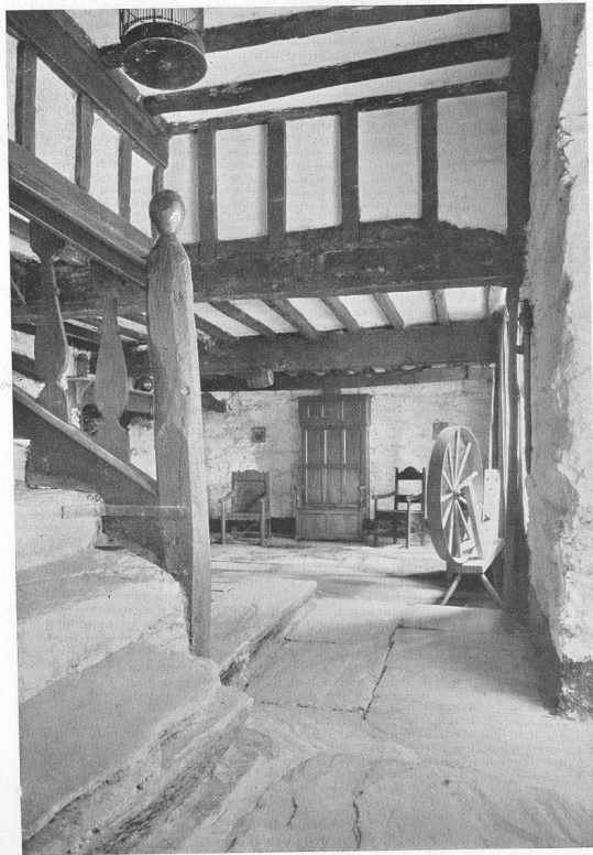
9.—STAIRS DOWN TO THE BREWHOUSE.
