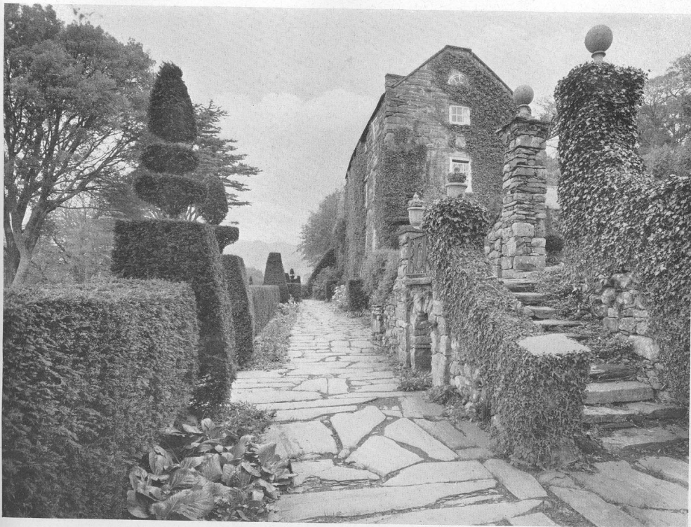
3.—THE SLATE-SLABBED TERRACE BELOW THE FORECOURT, AND THE CHARLES II WING.
